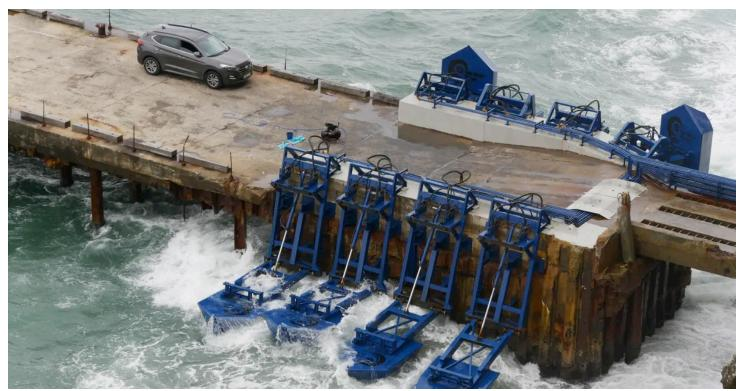
Some wave technology, like this one from Eco Wave Power, is deployed near shore, attached to seawalls or jetties, where paddle-like devices are driven up and down by wave action, activating hydraulic energy. Photo courtesy of Eco Wave Power
